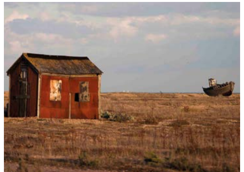
A long abandoned fishing hut sits on the shingle at Dungeness.
